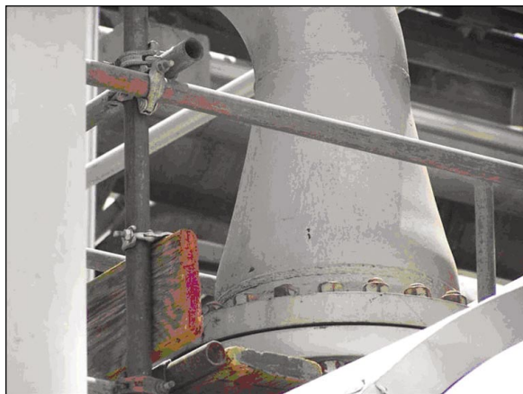
Fig. 1a (left) shows a general view of the selected 20-in. x 12-in. reducer; Fig. 1b shows the fiber-optic sensors attached on the reducer.
