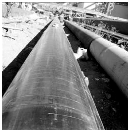
Pipeline operators may choose serpentine (photo above) or hoop (photo below) applications of fiber-optic sensors, among others, depending on the needs of the particular project (Fig. 4).
