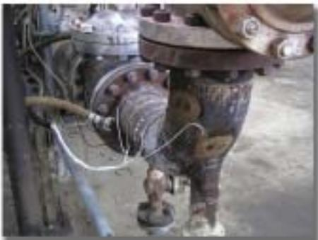
Fiber optic sensors rest on the exterior of the elbow section of an Alberta refinery pipeline to monitor telltale signs of corrosion. Courtesy of FOX-TEK.
